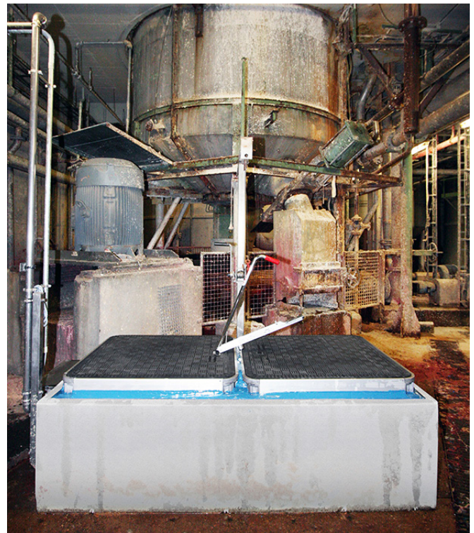
Complete installed Fibrelite covers
