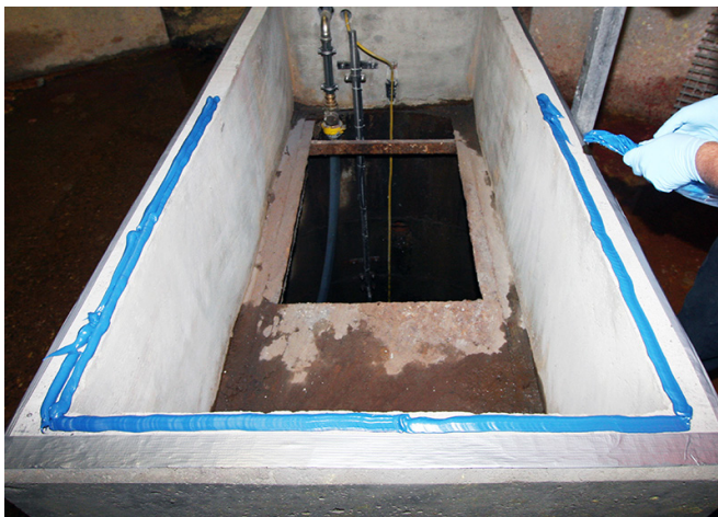
The blue epoxy resin is applied to the base
