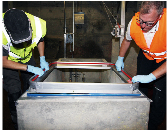
The aluminium frame is placed on the resin.
