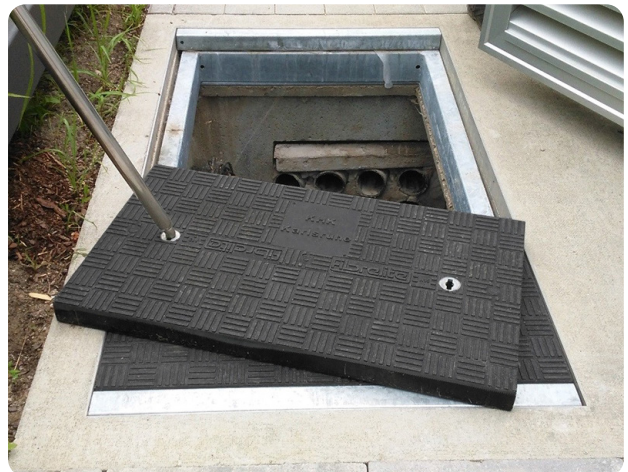
Fibrelite trench panels installed over the chamber
