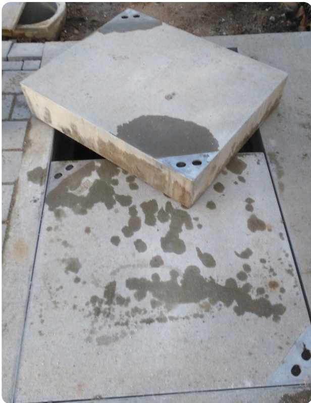
The original steel and concrete covers with a depth of 17cm
