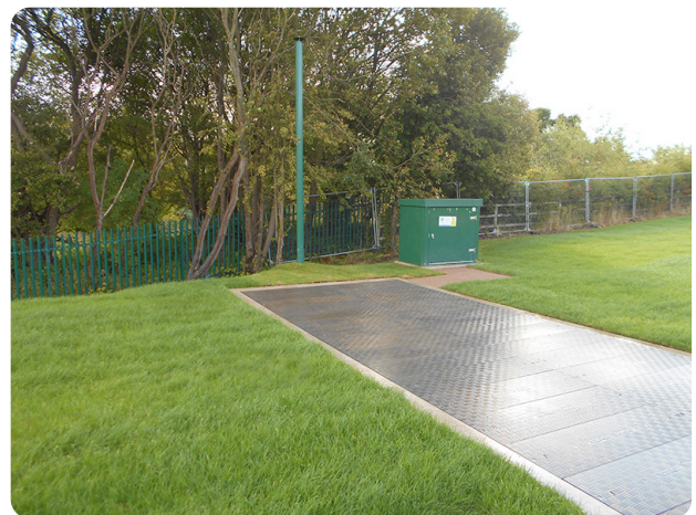
Each Fibrelite cover installed at this site is lockable for added security
