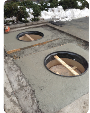
Fibrelite installations are simple – a fiberglass skirt can be used as a preform and to set the frame at grade
