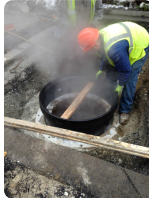
Fibrelite installations are simple – a fiberglass skirt can be used as a preform and to set the frame at grade
