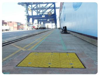
The Fibrelite 90 tonne load rated lightweight trench covers in position on the auavside
