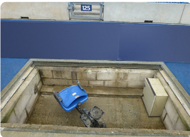
An existing camera pit to be covered by Fibrelite's composite trench covers
