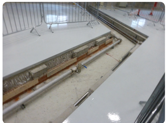
Complex corner trench design
