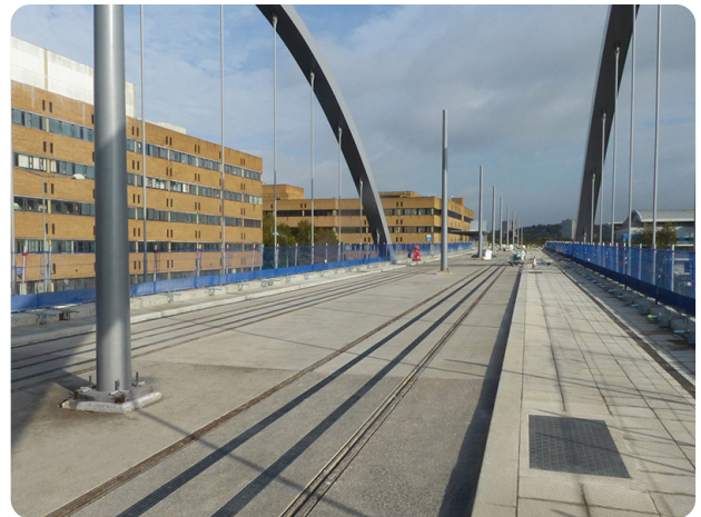
Fibrelite covers needed to be manufactured to work with pre-installed chamber systems
