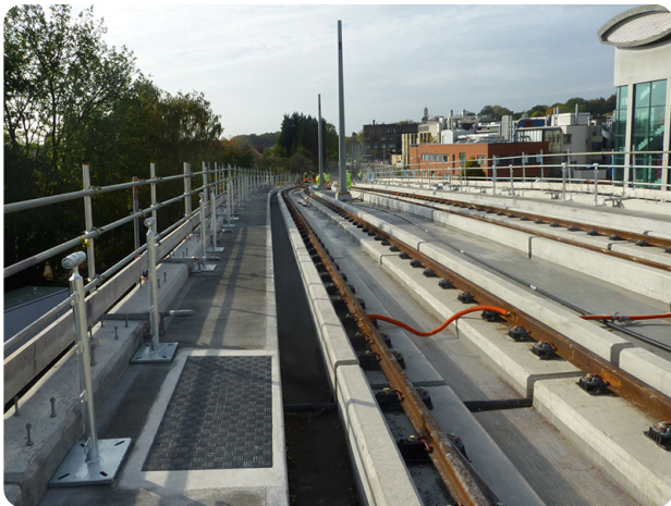
The Fibrelite B125 (12.5 tonne) load rated medium duty trench access covers
